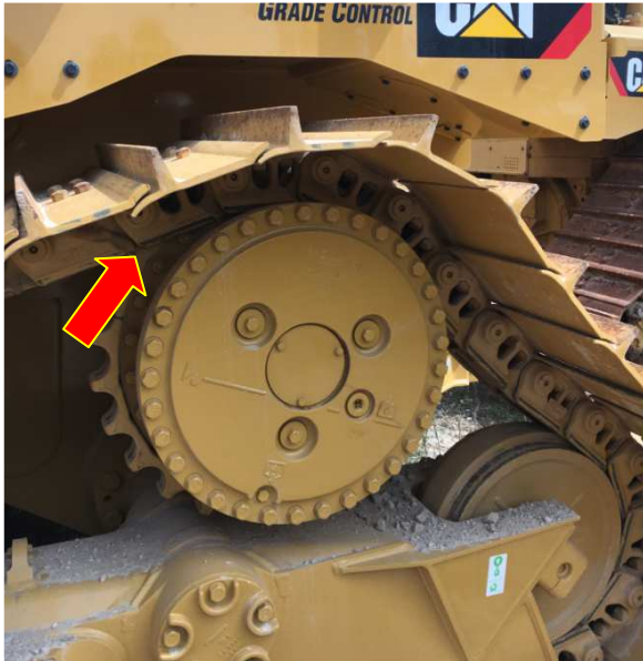
Fig. 2: Critical steel track wear point of a Track Type Dozer
